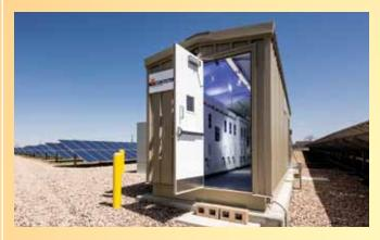
in the RPS Station, Bonfiglioli inverters are a climate-controlled plug-and-play solution for any environment and are covered by rapid, localized support and a warranty up to 20 years.
