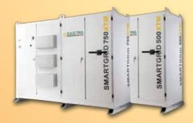
control and voltage and frequency ride-through. Listed to 1000 VDC, with a CEC weighted efficiency of 98 percent, the SGI 500/750XTM inverters set a new standard for large scale power conversion, says the company. www.solectria.com
