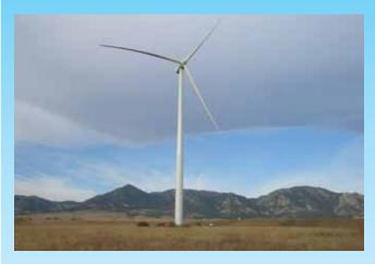
The G-97-2.0 MW Class IIIA wind turbine is Gamesa's answer to the growing demand for technological solutions that guarantee higher output at sites with low and medium wind speeds. The G97-2.0 MW features a swept area 16 percent larger than its predecessor and exceeds the energy output by nearly 14 percent. The model also features a new aerodynamic blade profile for maximum energy production and reduced aerodynamic loads on the nacelle.
