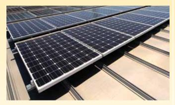
High strength-to-weight rail design keeps costs low while allowing for long spans up to 12 feet, says the company. The Renusol VS rail, approved for side mounting of WEEBs and grounding, saves valuable real estate on the top of the array and gives a cleaner look to the final solar installation.
