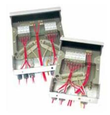
circuit inputs. The OutBack Power FLEXware series features rainproof, powder-coated UL-type 3R aluminum chassis, easy wiring configuration, and dual output lug terminals for up to 2/0 AWG conductors. www.outbackpower.com
