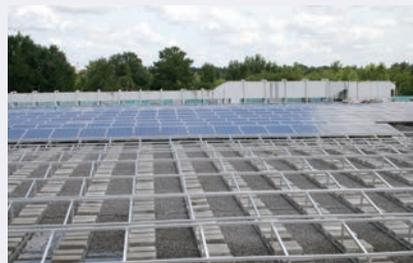
a ground mount solution. The SunRail system utilizes minimal parts yielding a fast, easy, and cost-effective solution for utility, commercial, and residential projects.
