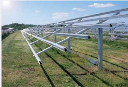
With a pile-driven galvanized steel post as its foundation, the system can reach installation times
