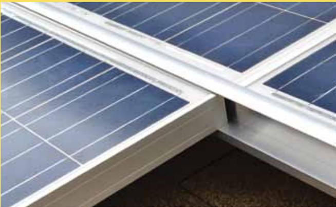
tems. Resting securely in place without clamps, modules are able to contract and expand naturally, minimizing the risk of micro-cracks and early module degradation. Finally, straight rows are automatically produced by the insertion rail, creating a continuous, even surface and a gap-free appearance.
