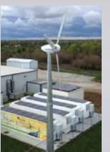
innovative approach to reduce stress on power plants and increase the reliability of electricity in industrial, commercial, and residential settings. EaglePicher's patented Power Pyramid hybrid solution, which utilizes a multitiered battery system, can provide the necessary flexibility and modularity to control and regulate renewable energy.
